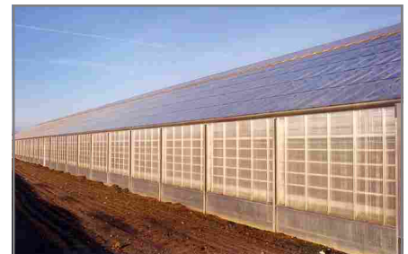
Polycarbonate sidewalls and glass roof top
