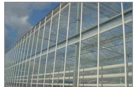
Sidewall roller screens
