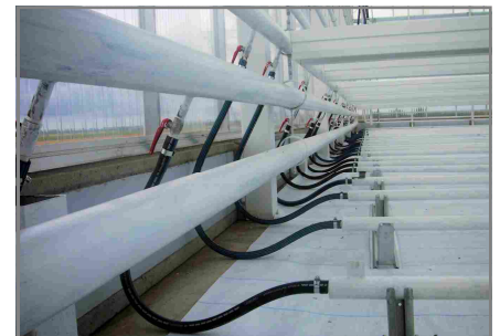
Distribution with Tichelmann system
