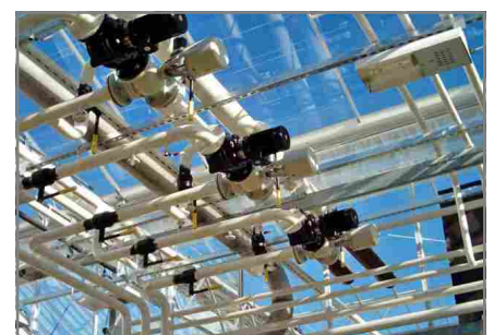
Mixing stations placed over path
